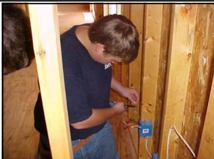
Electrical Technology student, Bradley Stoker, is wiring an outlet.
